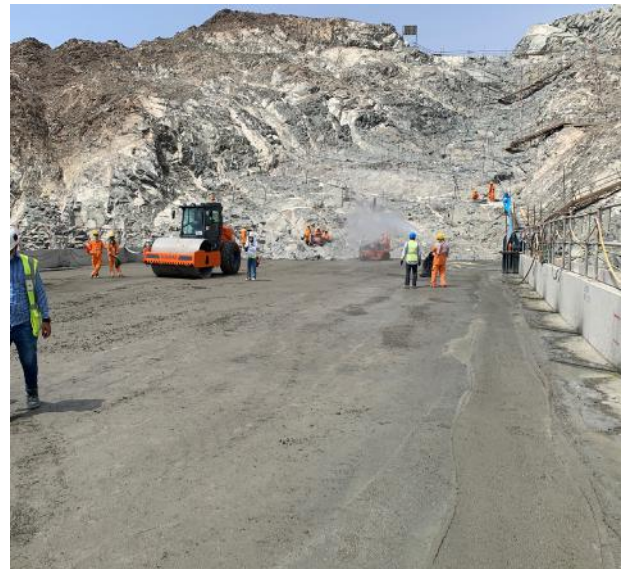
Installation work in progress
