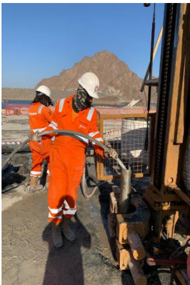
Standpipe piezometer installation
