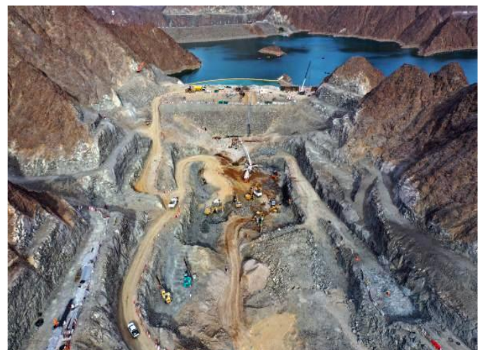
HP Tunnel Portal Upper Intake
