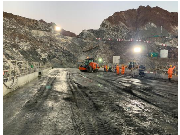
Saddle Dam during construction
