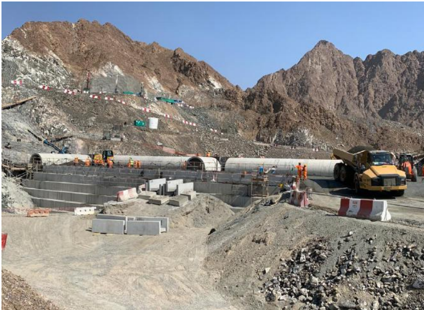
Construction works in progress
