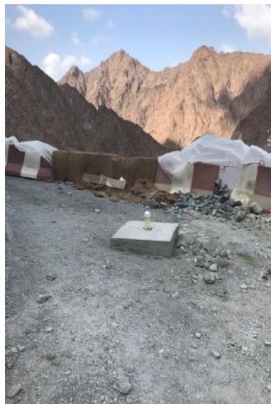
Inclinometer installation
