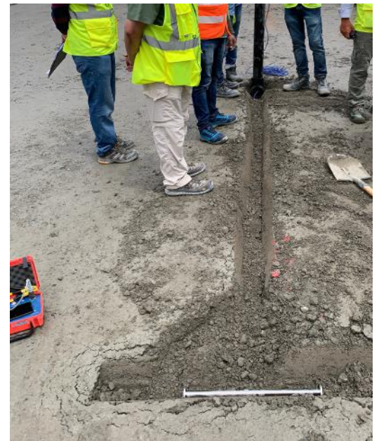
Strain gage (LBSGTM) installation
