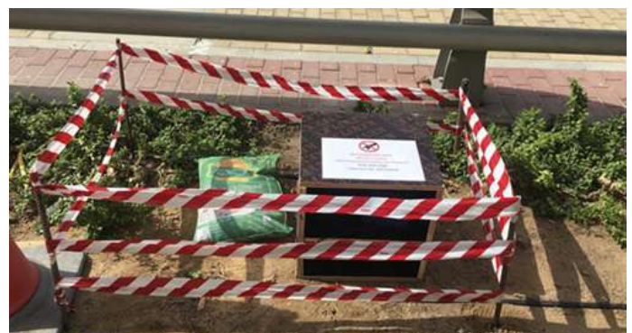
Vibration monitoring near tram alignment
