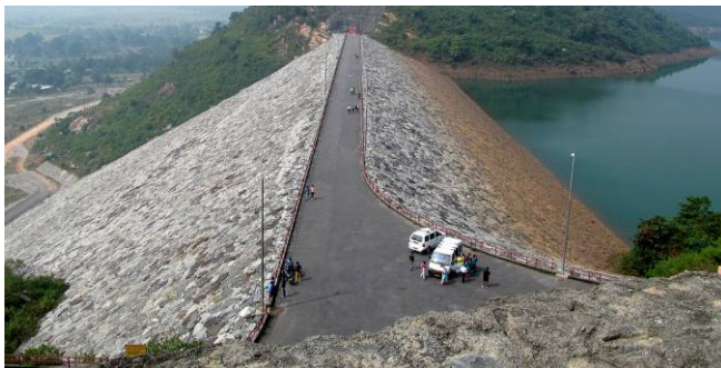
Purulia earth dam, India
