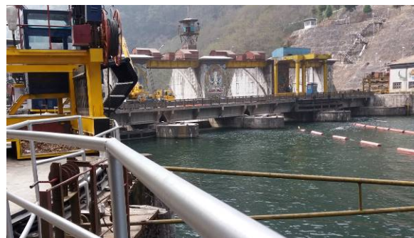
Chukha concrete gravity dam, Bhutan
