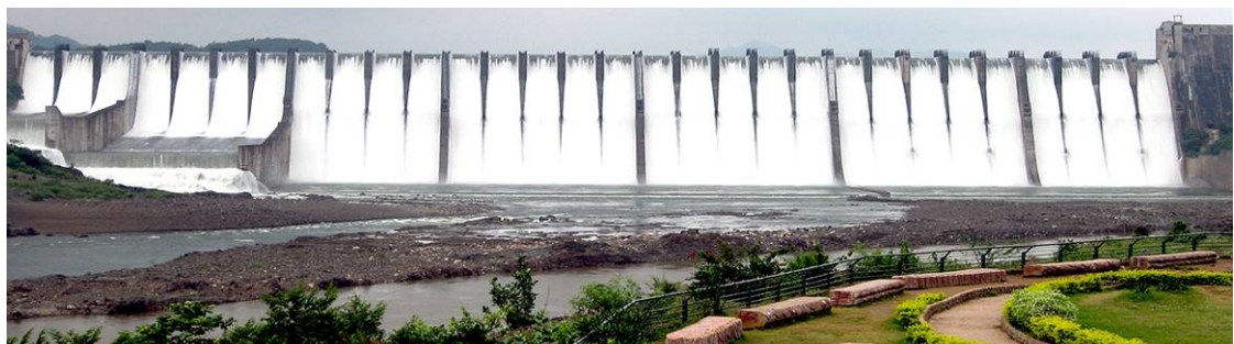
Sardar Sarovar concrete gravity dam,
