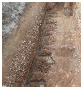
Settlement cell being installed at Gibe III dam, Ethiopia
