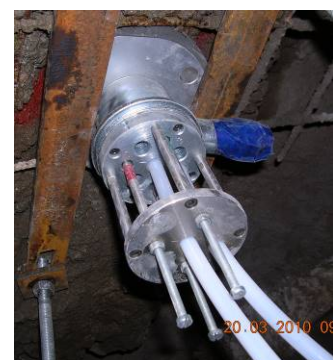
BHE and load cell in powerhouse at Koprubasi HEP, Turkey
