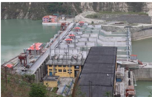
Teesta concrete gravity dam, India
