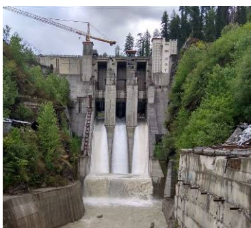
Parbati concrete gravity dam, India
