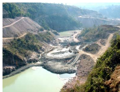
Work in progress at Kol earth dam, India
