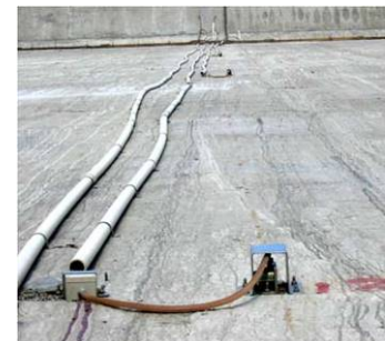
Tilt meter installed at concrete face of Dhaultiganga CFRD, India
